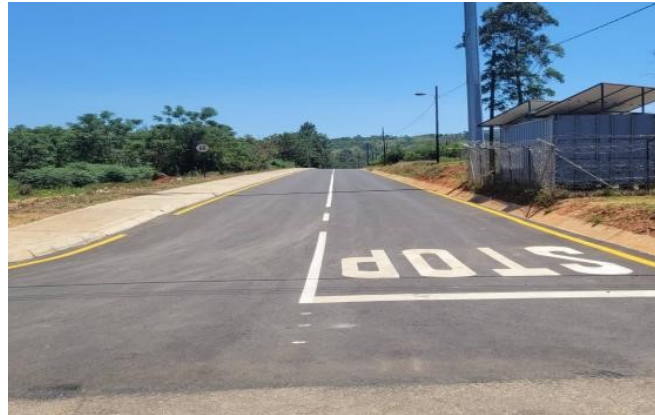
Completed Titandini Road
