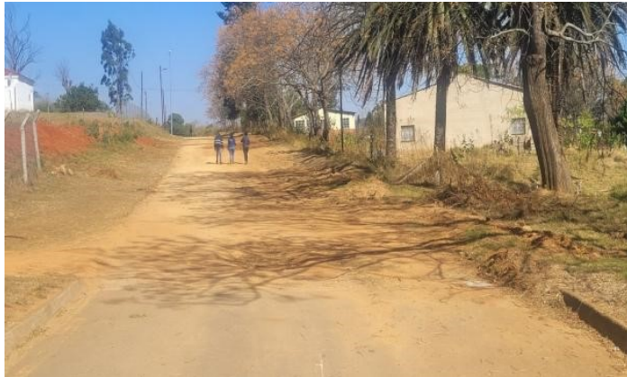
Titandini Road before construction
